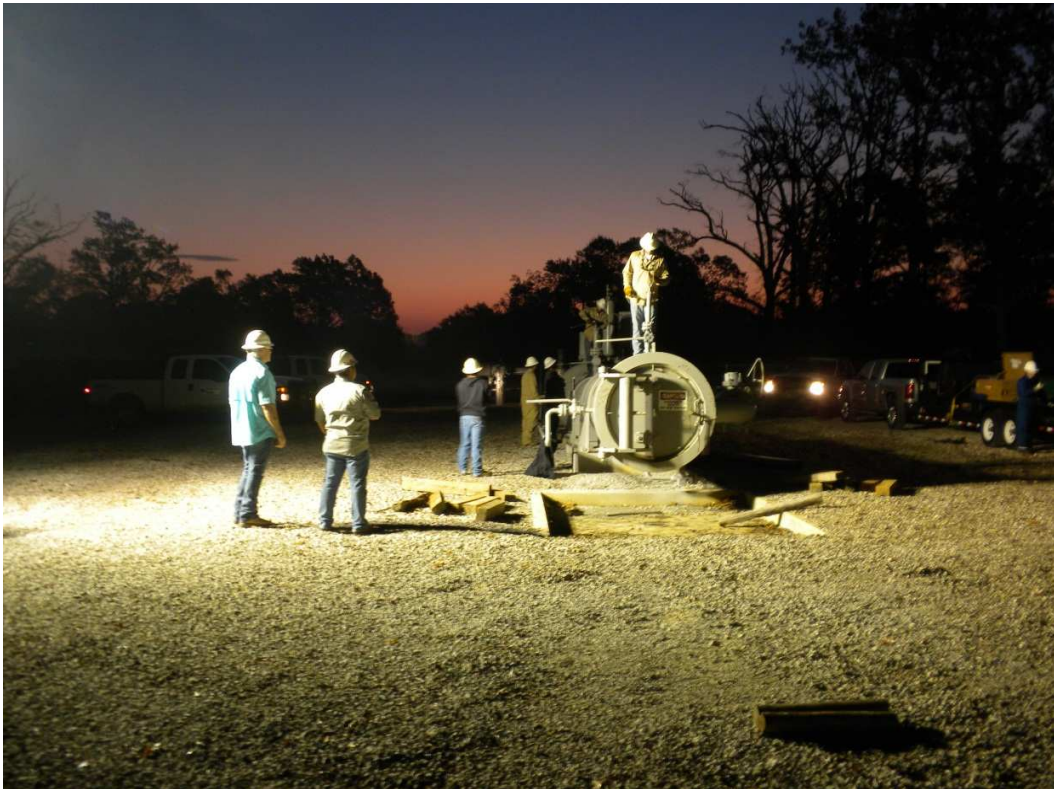
Figure 1: Coordinating plans to launch a pipeline cleaning tool
